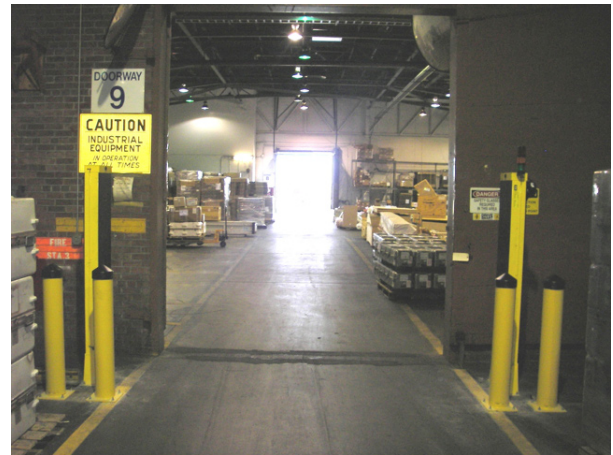
Figure 2: ATAC Choke Point with RFID Portals
