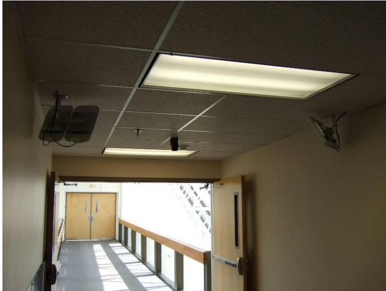
Figure 16: Picture - MSU Bridge 1
