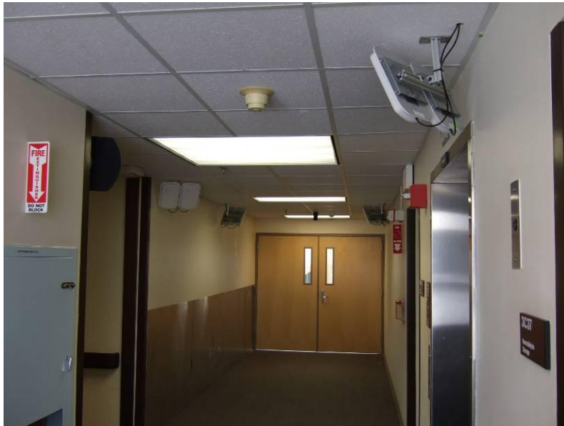
Figure 17: Picture - MSU Bridge 2
